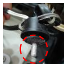
Thermistor get stuck by lint, and residue
