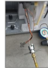
Picture Checking Flow Through Capillary Tube
