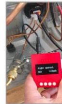
Picture Checking Flow with 3-way (Open Right)
